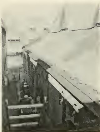
Figure 4 Roof over south side eave of sanctuary below clerestory dormers
